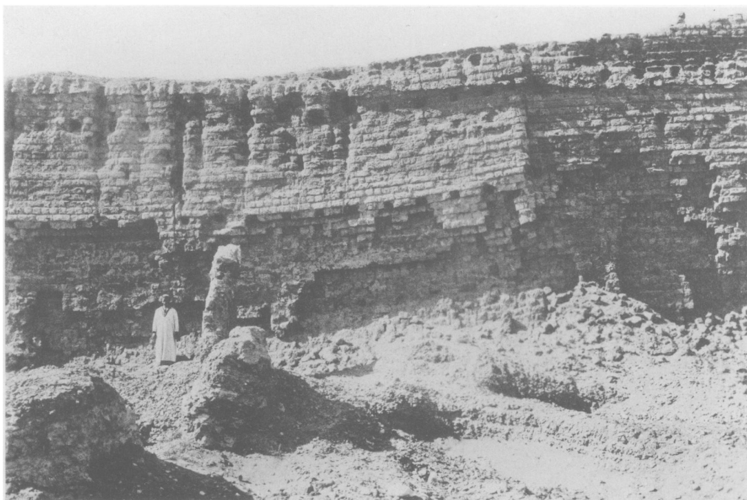
The West Wall, Inner Face
