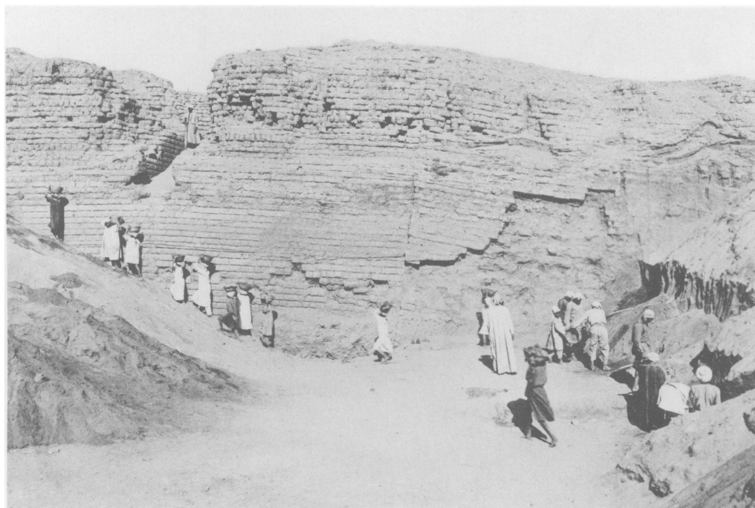
A Clearance of Sand from the North Wall, Inner Face
